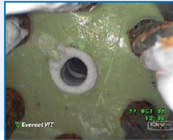
Anchor Close-Up, Top of Tendons Show Corrosion
