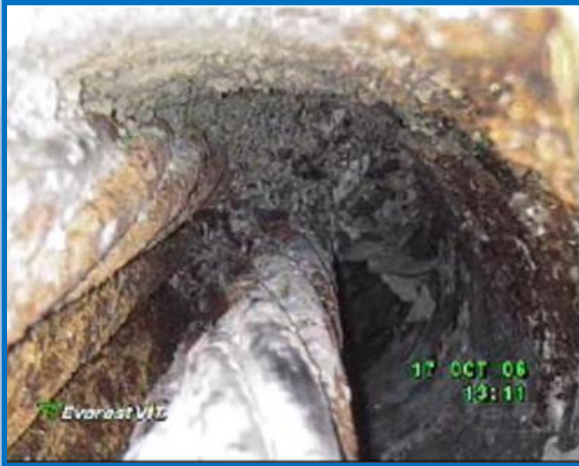
Void Bottom Corrosion on Duct & Tendons
