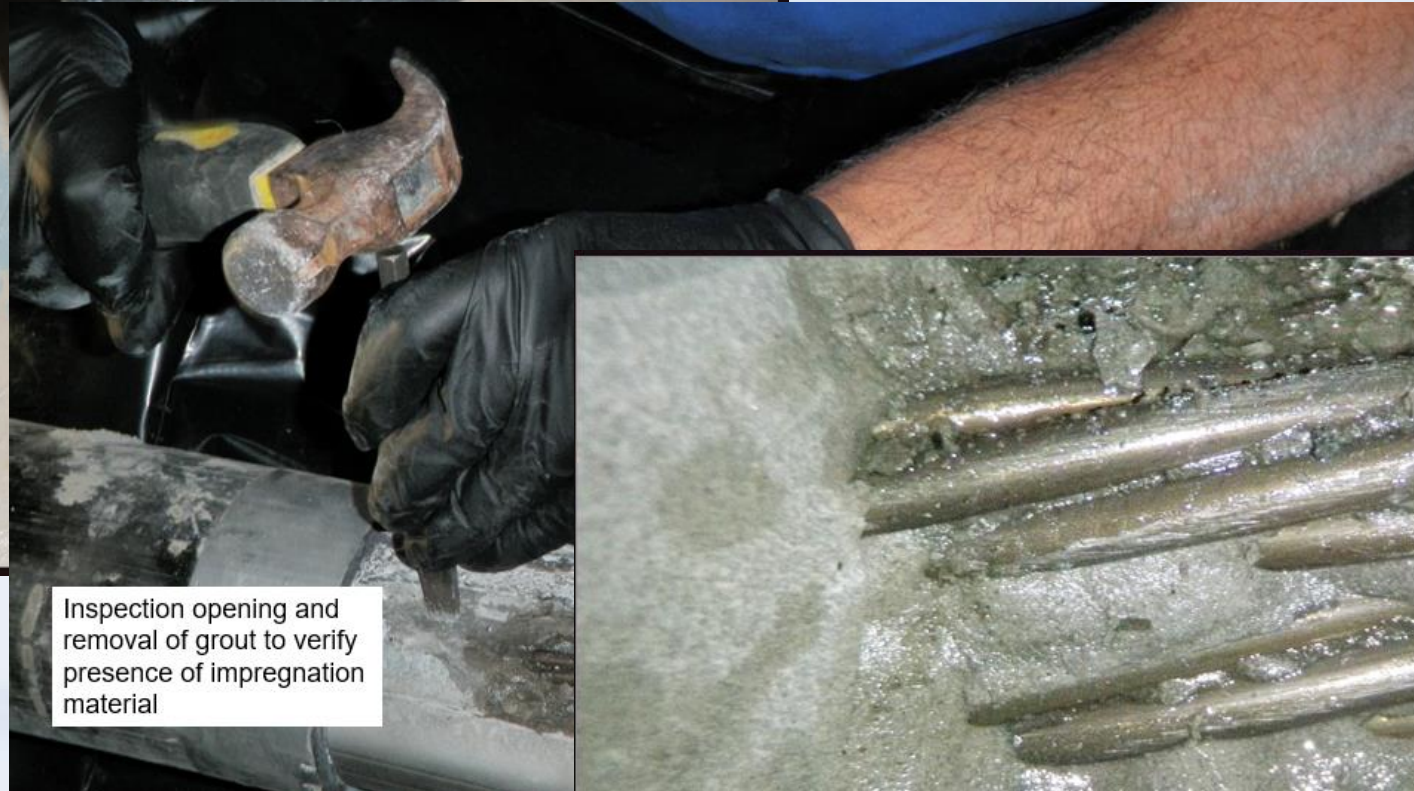
Impregnation material visible along all PT strands
