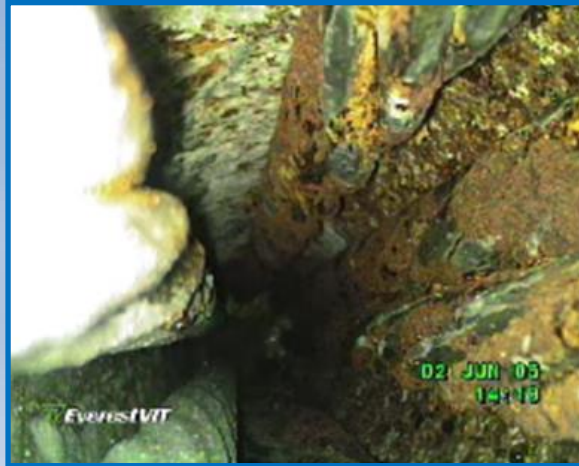
Corrosion on Duct & Tendon
