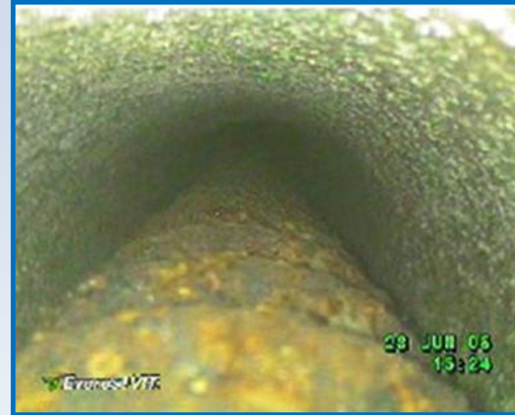
Void in Pier With Dywidag Bar Instead of Tendons
