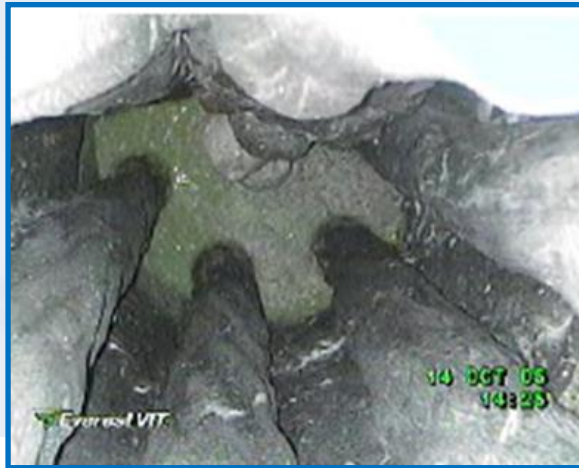
Anchor Plate, Tendons & Duct are Grout Coated
