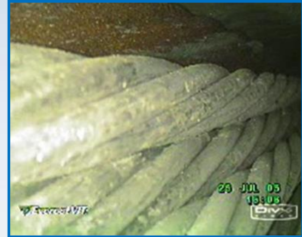
Corrosion on Duct
