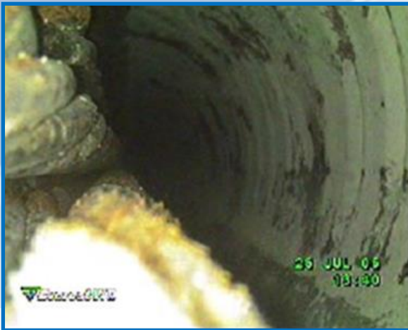
Void With Tendon Corrosion
