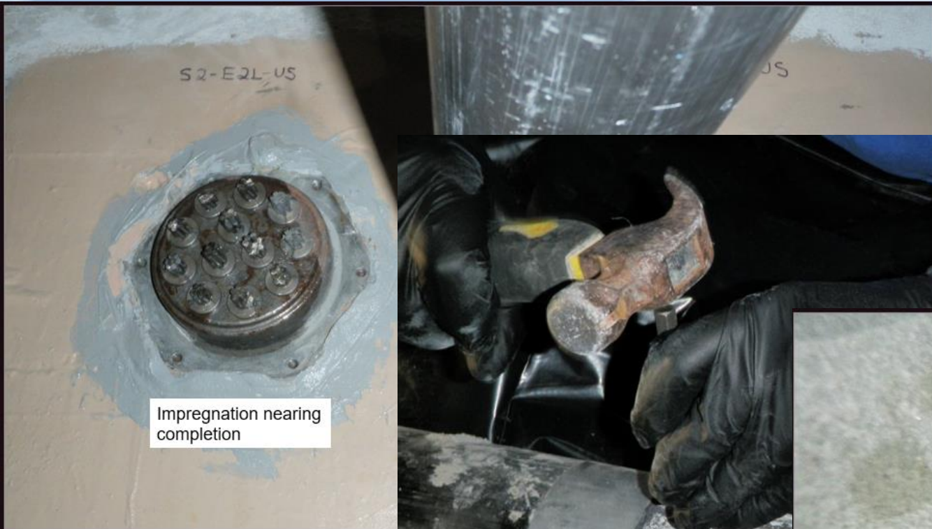
Inspection opening and removal of grout to verify presence of impregnation material
