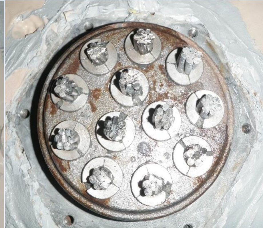
Exposed Strands after Grout Removal
